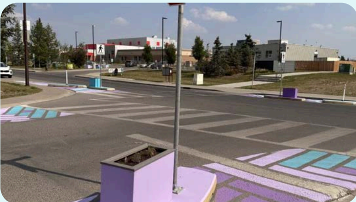
Curb extension & pavement markings. Credit: ActivateYYC
