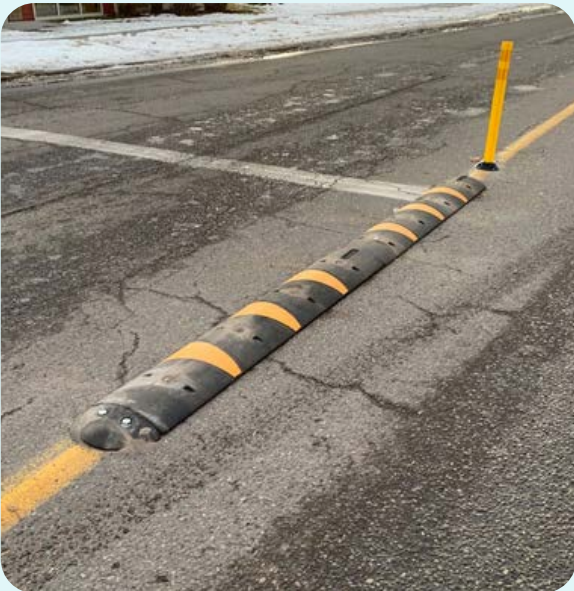
Speed hump. Credit: City of Calgary
